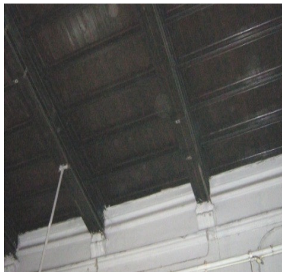
Figure-17 Mahogany wood ceiling with molding to enhanced the design in the Raj Bhawan
