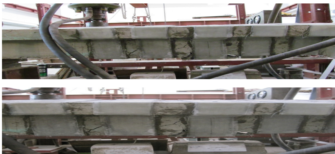
Figure-6 Beams retrofitted with Fully-wrapped GFRP oriented at 90°
