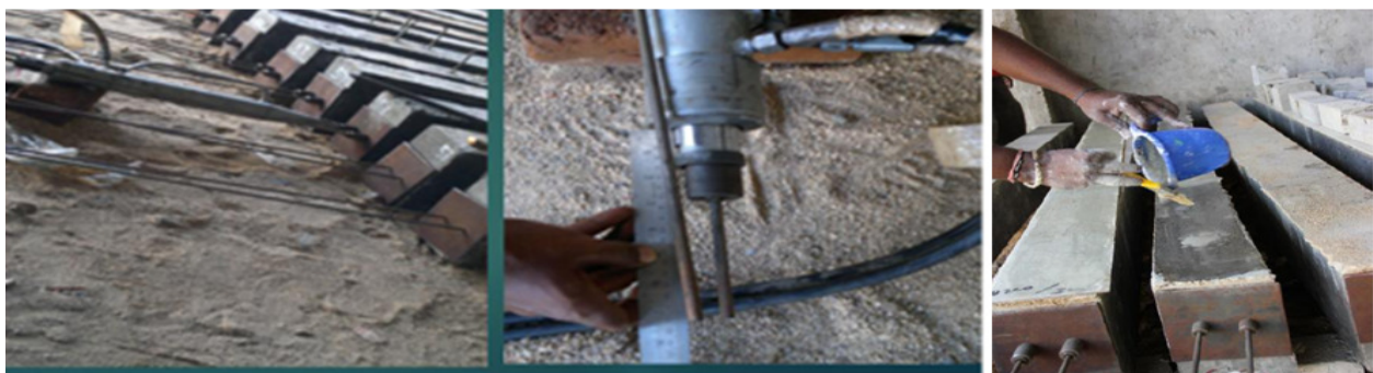
Figure-2 Stressing the prestressing wire and application of FRP on beams
