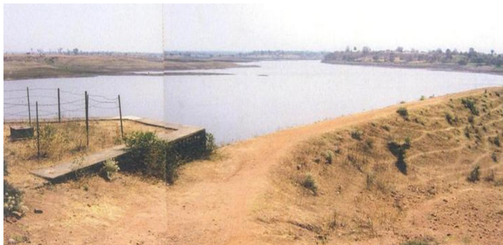
Figure-2 Panoramic view of Mod sagar reservoir of Jhabua District
