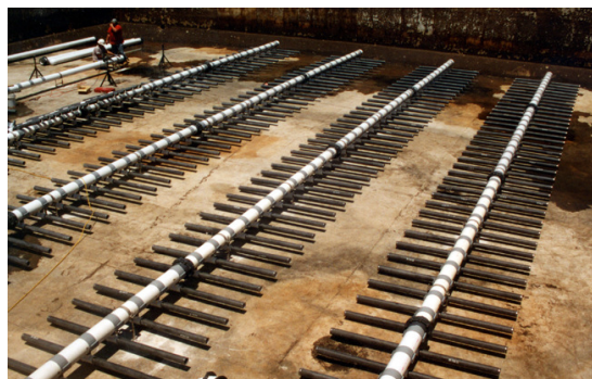
Figure-1 Diffused Aeration System
