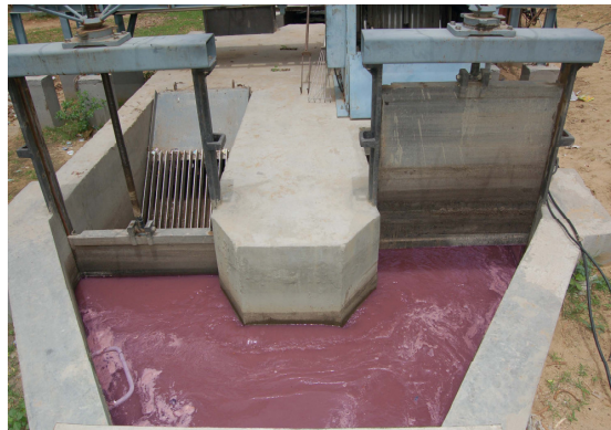
Figure-3 New Coarse Screen
