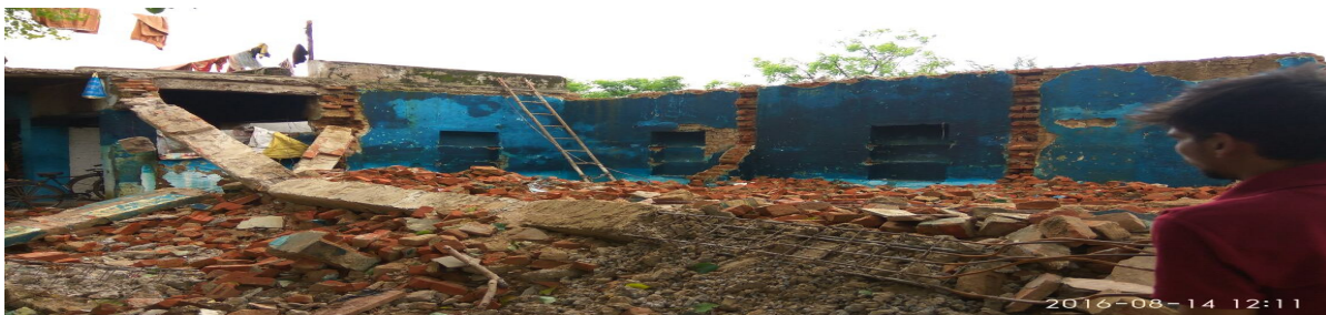
Figure-1: Site at Moudapara, Raipur showing debris of demolished structures.
